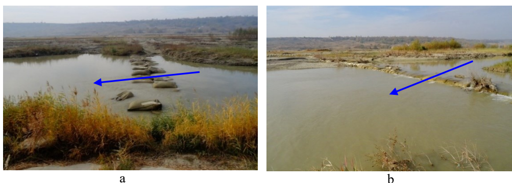
Fig. 6. Calibrated Moldova River bed bottom sills degradation stages: a - geo-bags displacement the from the bottom sills; b - downstream view of the bottom sill (year 2018).
